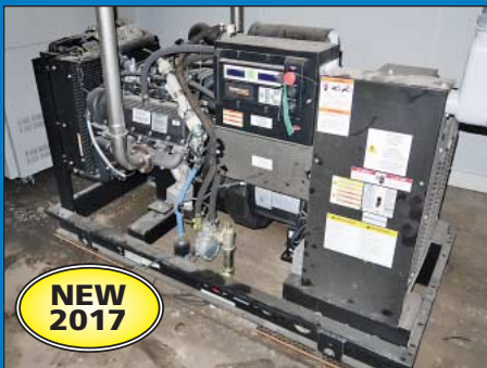
50 KW Generac Model SG50 Natural Gas Powered Generator Set
