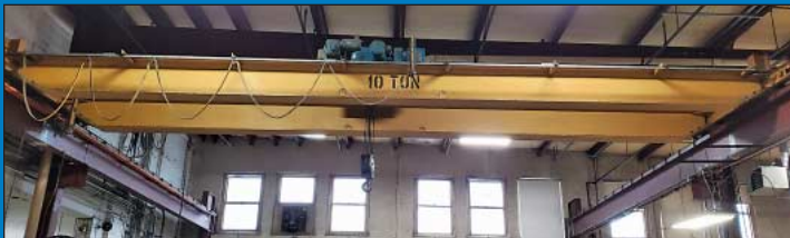
10 Ton X 42' Span (Approx.) Progressive Double Girder Top Running Overhead Crane
